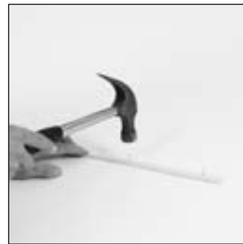
Take the piece that was snapped off earlier and mark the positions of the wires with a pen. Tap three nails in.
